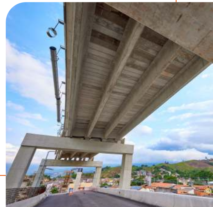
Caraguatatuba and São Sebastião Road Bypasses Caraguatatuba and São Sebastião / SP
